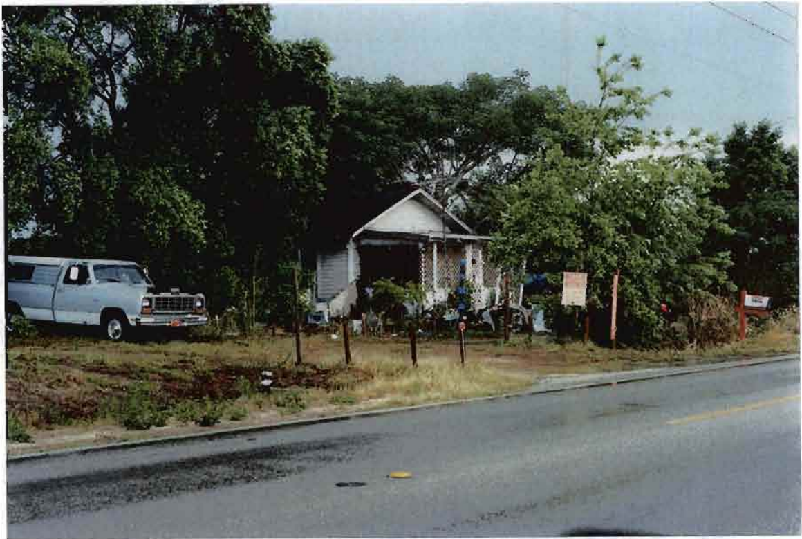
Deteriorated Building & Site.
