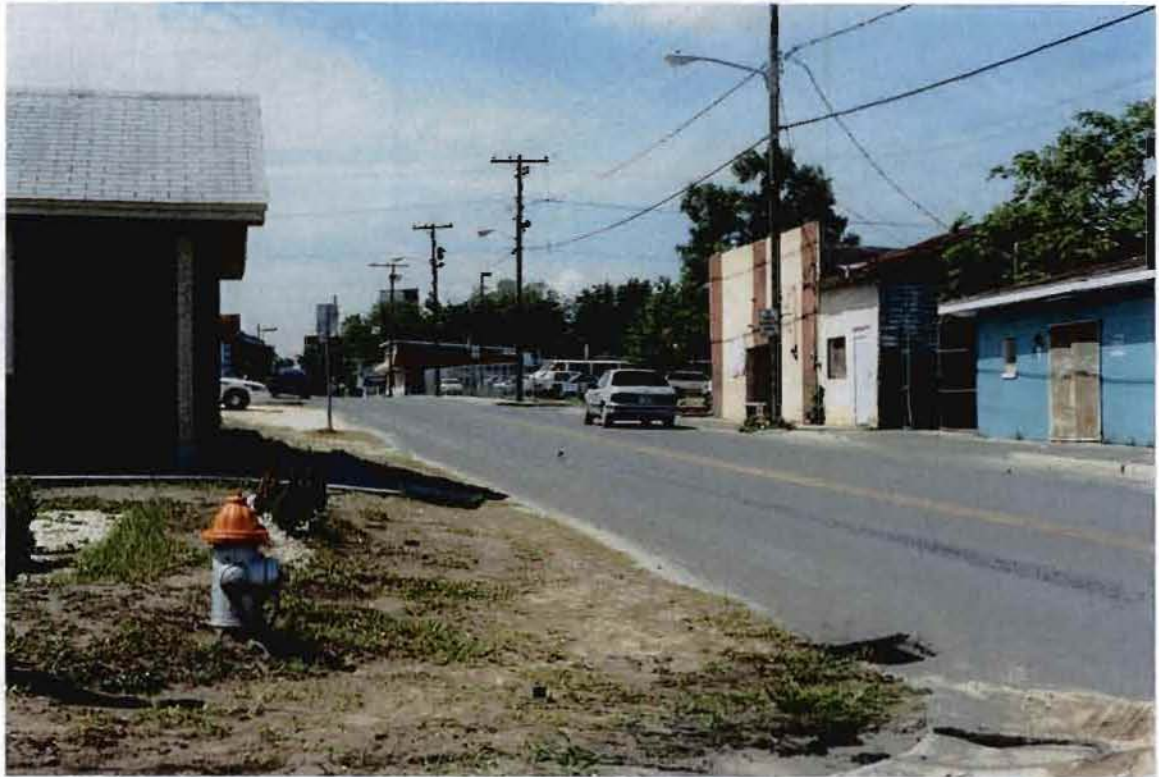
Defective Street Layout, Faulty Accessibility/Usefulness, Unsafe Conditions, Deteriorated Building & Site, and Deteriorated or Hazardous Conditions.
