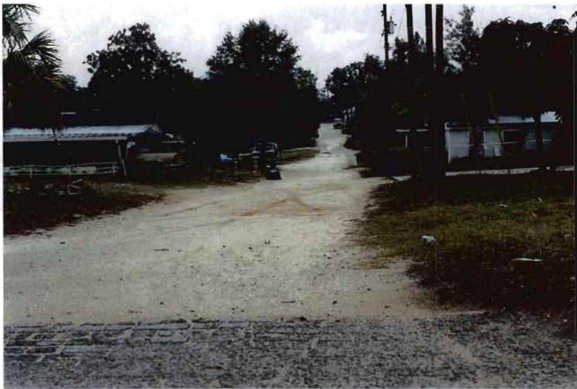
Faulty Accessibility/Usefulness & Deteriorated or Hazardous Conditions.
