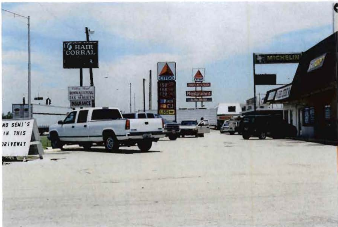
Defective Street Layout, Faulty Accessibility/Usefulness, Unsafe Conditions, Deteriorated Building & Site, and Deteriorated or Hazardous Conditions.
