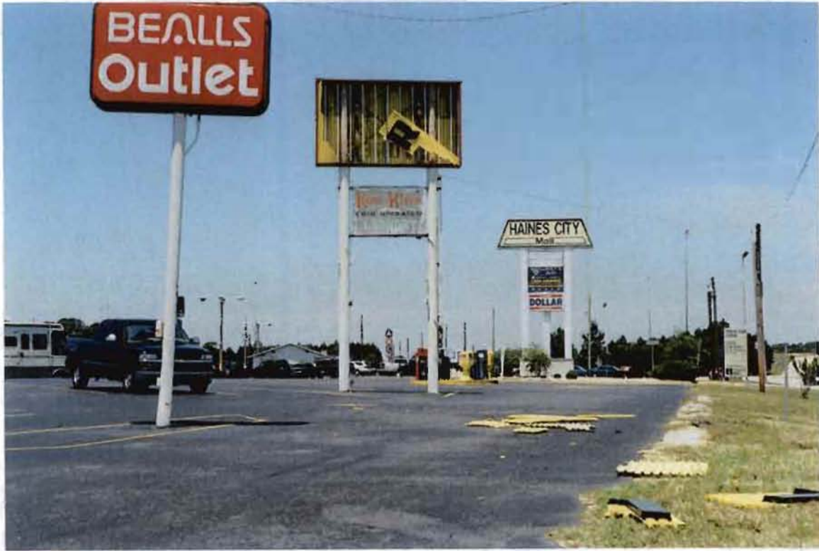
Defective Street Layout, Faulty Accessibility/Usefulness, Unsafe Conditions, Deteriorated Building & Site, and Deteriorated or Hazardous Conditions.
