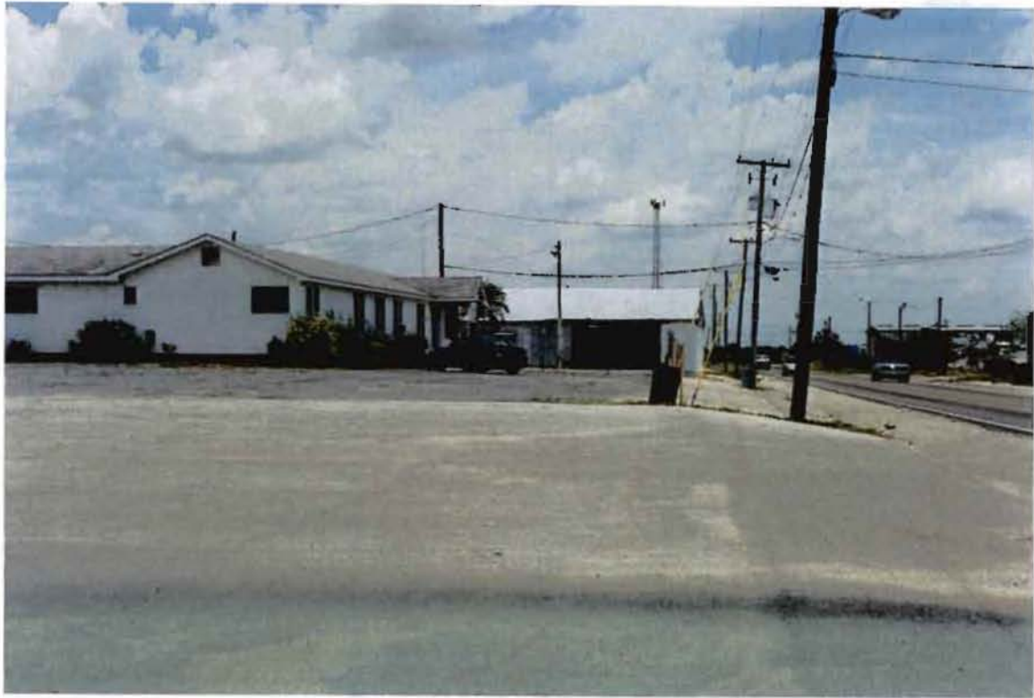
Faulty Accessibility/Usefulness & Deteriorated Building & Site.
