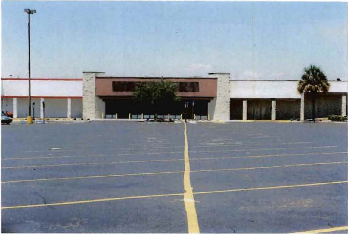
Deteriorated Building & Site.
