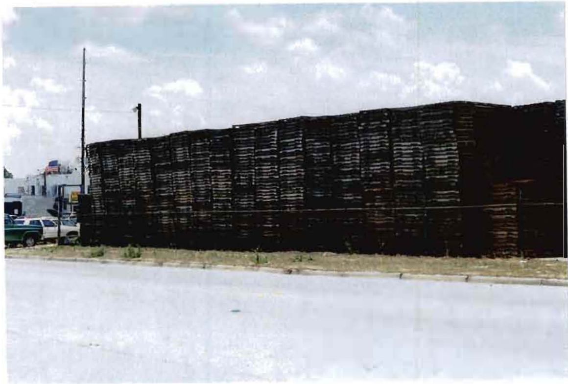
Deteriorated Building & Site, and Deteriorated or Hazardous Conditions.
