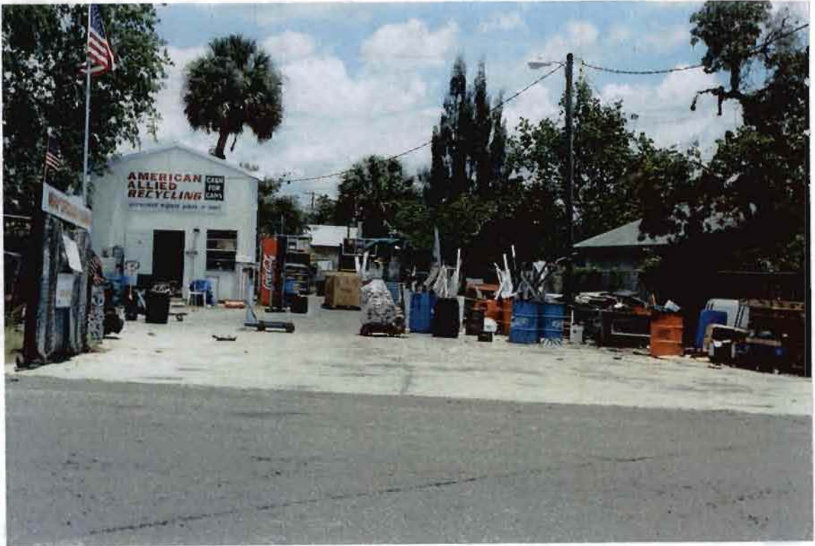
Faulty Accessibility/Usefulness & Deteriorated Building & Site.
