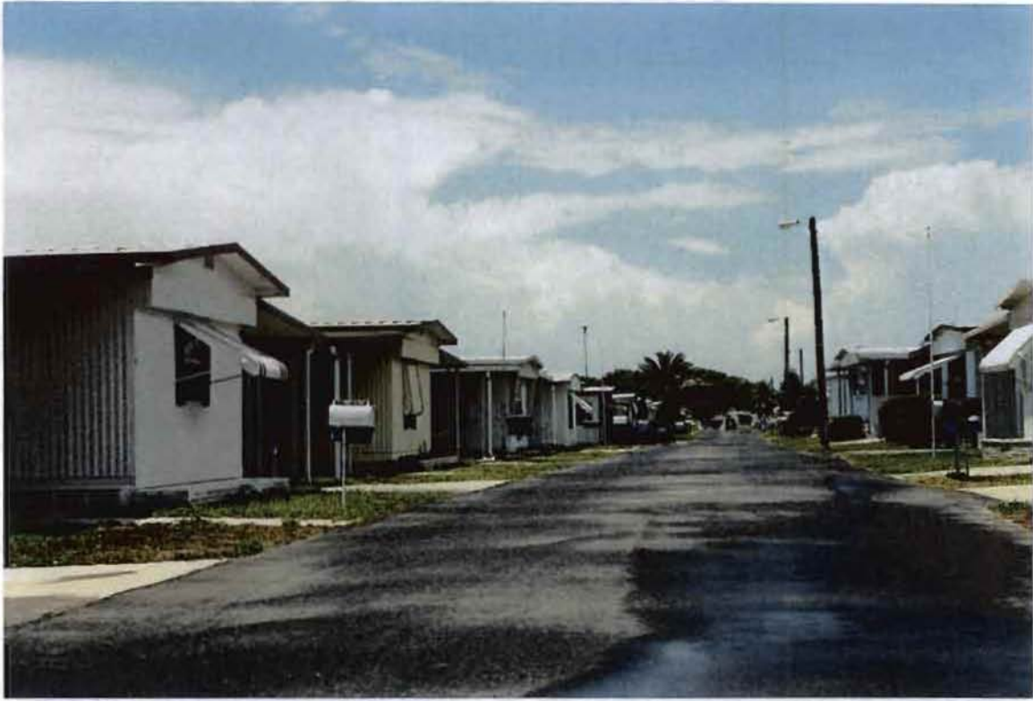
Deteriorated Building & Site.
