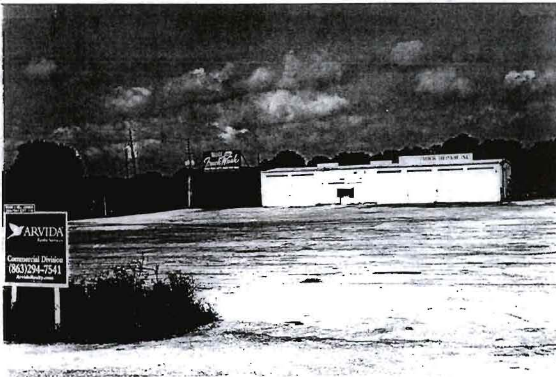
Defective Street Layout, Faulty Accessibility/Usefulness, Unsafe Conditions, Deteriorated Building & Site, and Deteriorated or Hazardous Conditions.
