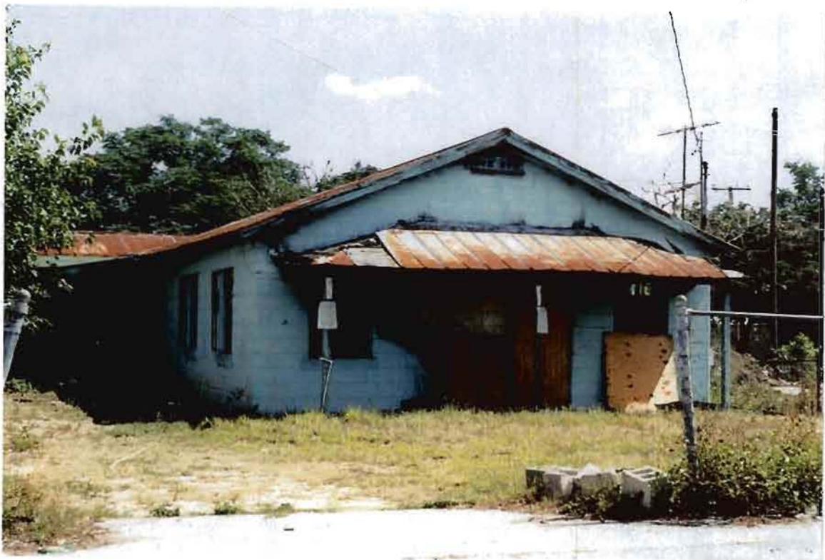
Deteriorated Building & Site.
