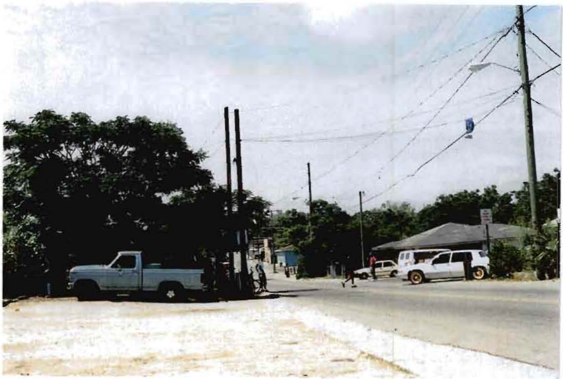
Defective Street Layout, Faulty Accessibility/Usefulness, Unsafe Conditions, Deteriorated Building & Site, and Deteriorated or Hazardous Conditions.
