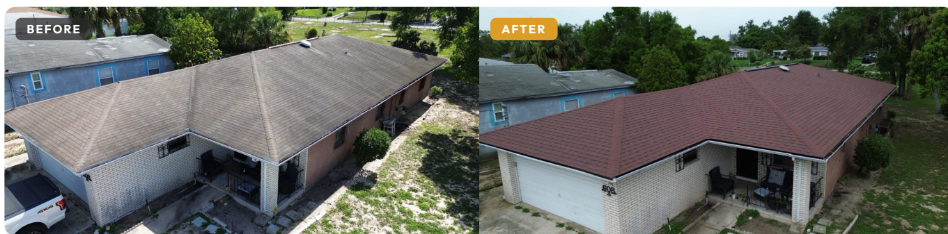
Full roof replacement — protection that matters most.
